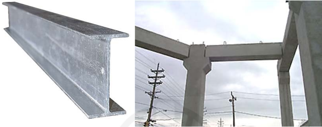
Figure 1-3: Steel and concrete beams
